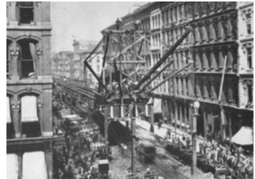
Elevated Loop Construction, 1895, Chicago.
