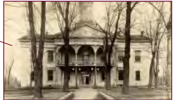
Illinois State Capitol, 1839, Vandalia.
